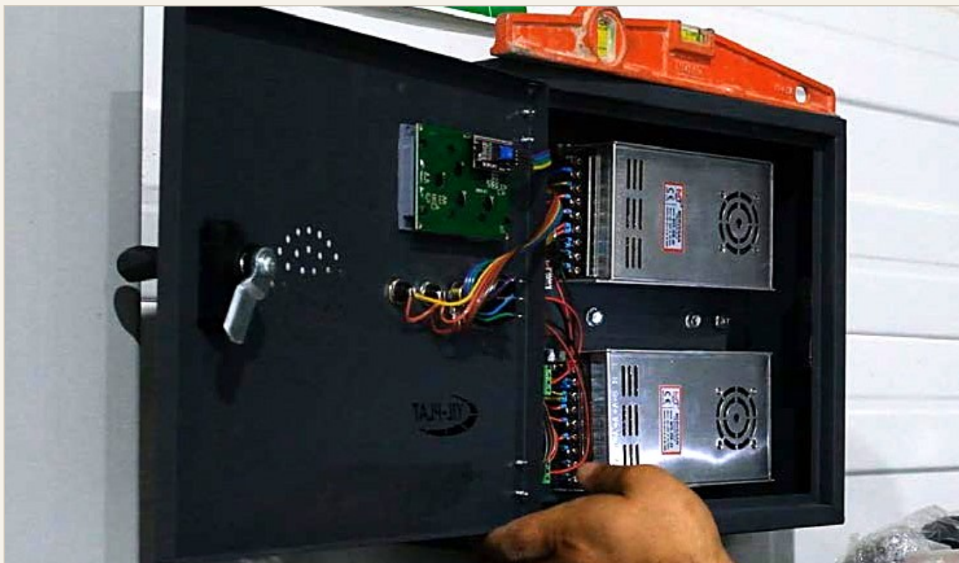
9A · THE PANEL LEVELLED AND OFFERED UP TO THE WALL
