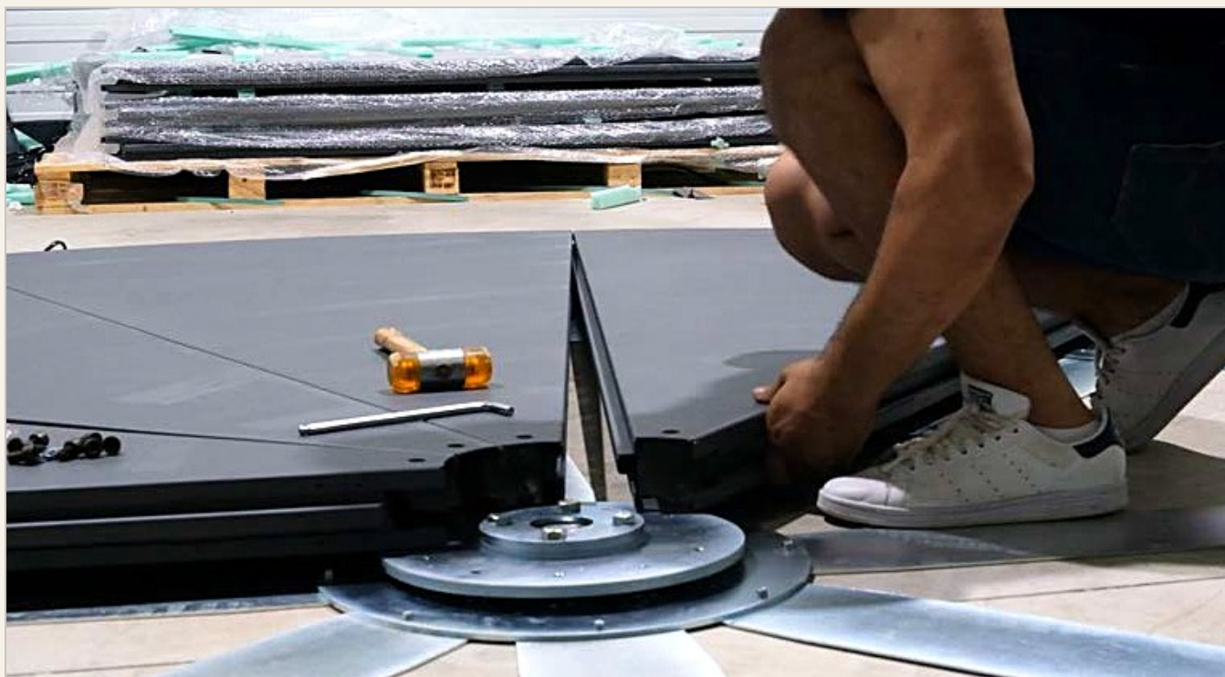
5C · THE FINAL PANELS DROPPED INTO SEQUENCE AROUND THE DECK
