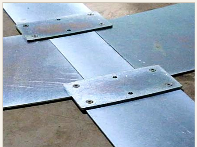
3B · INNER PLATES JOINED WITH CROSSHEAD SCREWS
