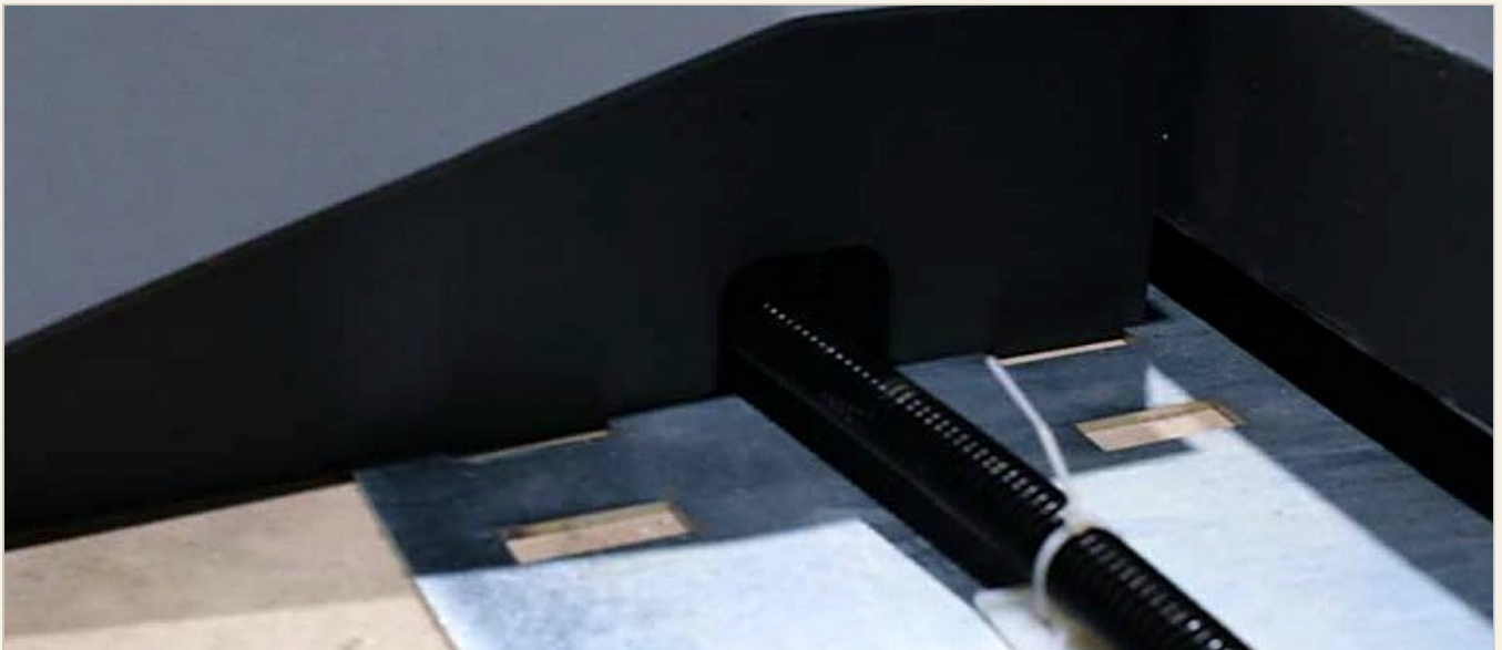
8C · THE SLEEVED CABLE SEATED IN ITS PASSAGE, NOTCHES ENGAGED
