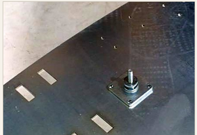
4B-I · WHEEL-SUPPORT STUD FIXED TO THE OUTER ARC
